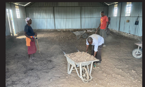
NEW BUILDING CONSTRUCTION
