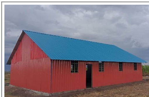
Church building under roof
